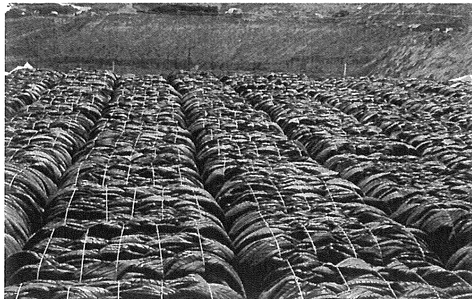
Using compressed, used tyres on the A421 improvement in bales turned was similar to laying bricks
